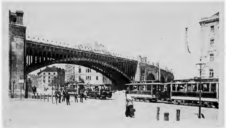
LXXVII. VIENNA. A RAILWAY VIADUCT PASSING OVER AN IMPORTANT STREET.
